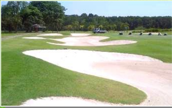
Repair & Uplift Bunkers at Hole #12
